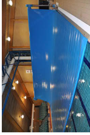
Figure 16 - Pool cover to be utilised on all pools to reduce evaporation and correspondingly save significant amounts of energy (courtesy of covers4pools)
