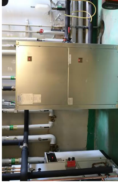
Figure 9 - Typical ground source heat pump of circa 60kW
